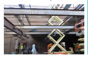
The New Gym is shaping up with structural steel and decking being placed in all areas this month. Concrete on the elevated decks at the New Gym area will be taking place this month, closely followed by MEP/F overhead rough in and fireproofing. The New Theater CMU walls and slab-on-grade concrete is in process this month. The New Kitchen/Commons slab-on-grade will pour towards the end of the month.
